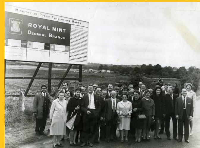
The site of the new Decimal Branch of the Royal Mint at Llantrisant.
